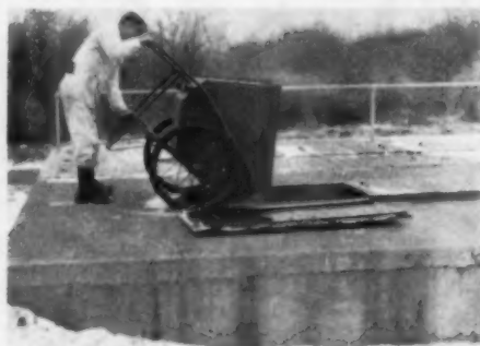
Fig. 2—The doors on the top of the manure pit.
